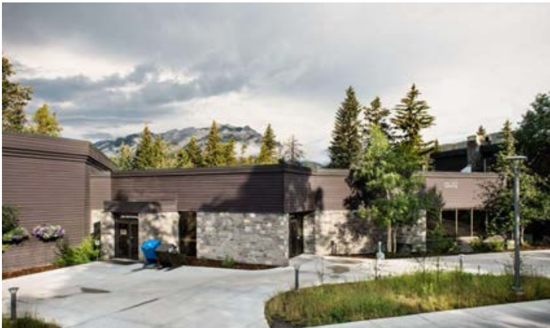
Max Bell Building Facing North (West) - Mount Norquay Photo by Don Lee, Banff Centre
